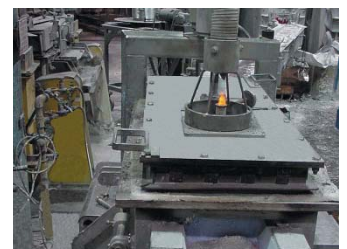
Fume exhaust system
