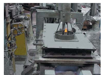
Fume exhaust system
